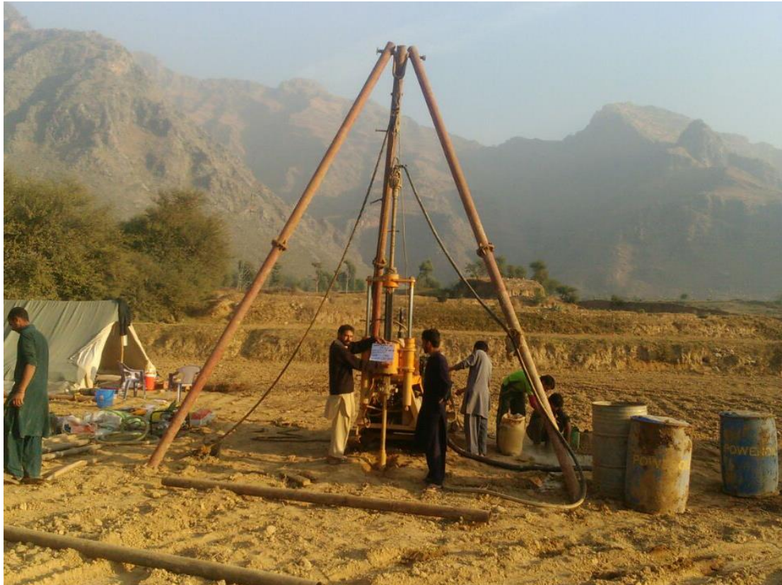
Geotechnical Investigations along the proposed Alignment of Swat Expressway
