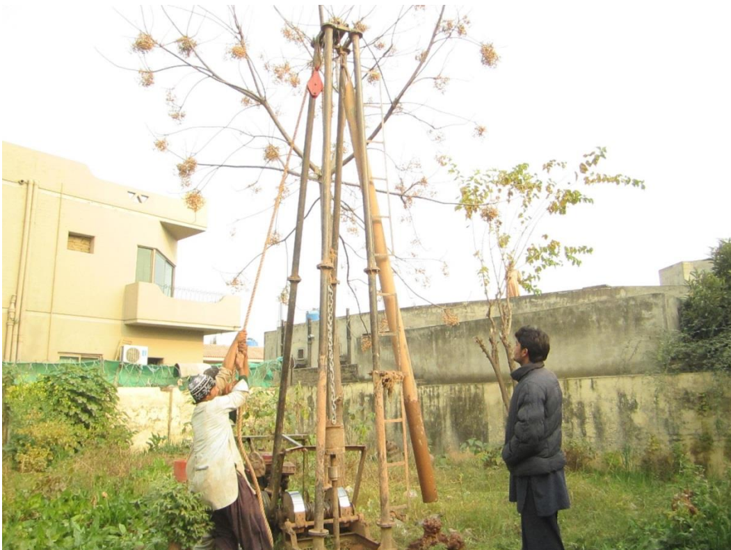
Geotechnical Investigations of Residential Building in Bani Gala, Islamabad
