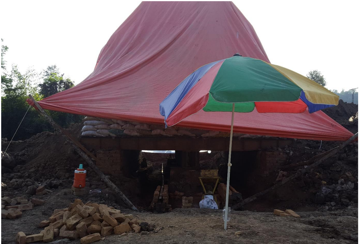
Pile Load Test at Tarar Campus, University of Poonch, Rawalakot, AJ&K
