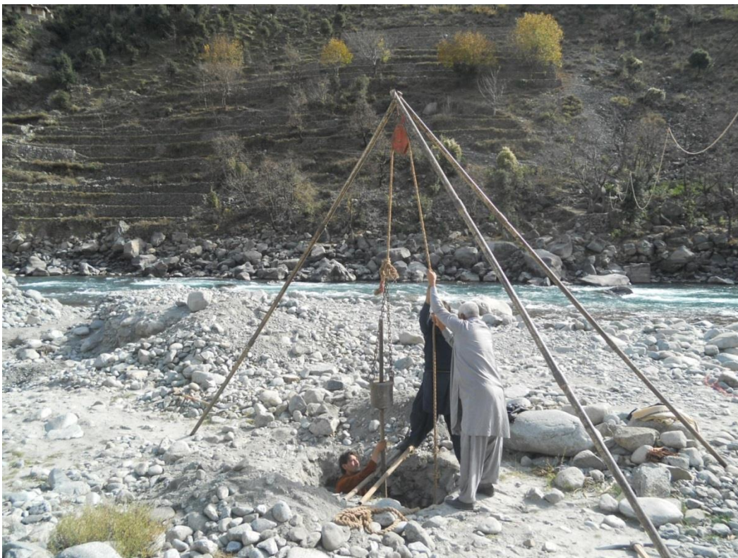
Geotechnical Investigations of Phunkia Bridge, Bahrain, District Swat, KPK
