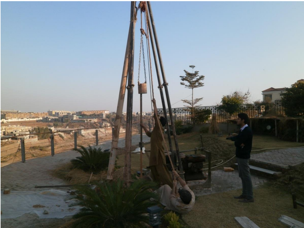
Geotechnical Investigations for Slope Remediation in DHA, Phase-II, Islamabad
