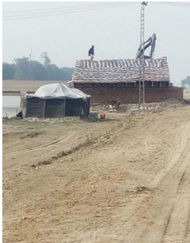
Static Pile Load Test at Ghotki
