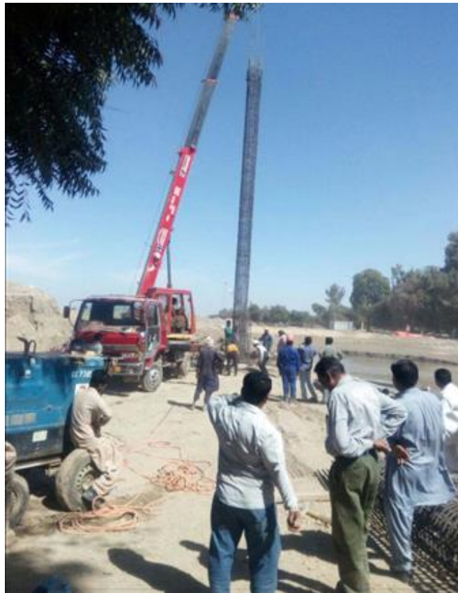
Piling Work at Ghotki
