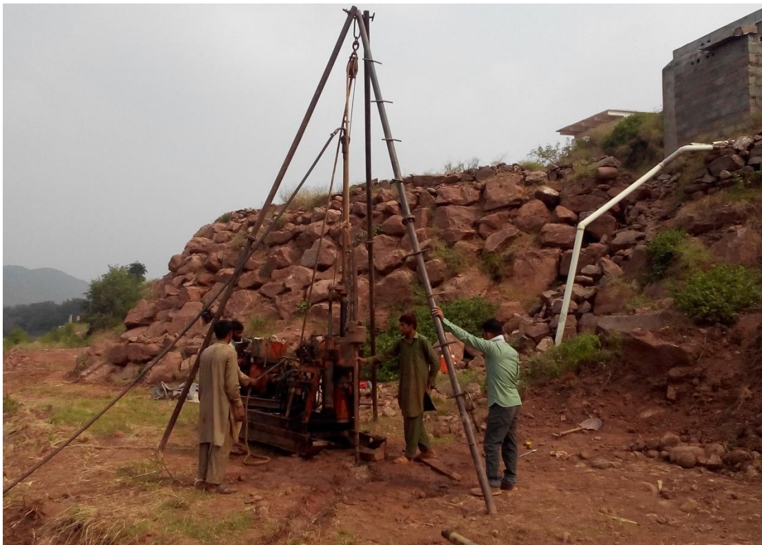
Geotechnical Investigations for M-3 Embankment in Bahria Golf City, Islamabad
