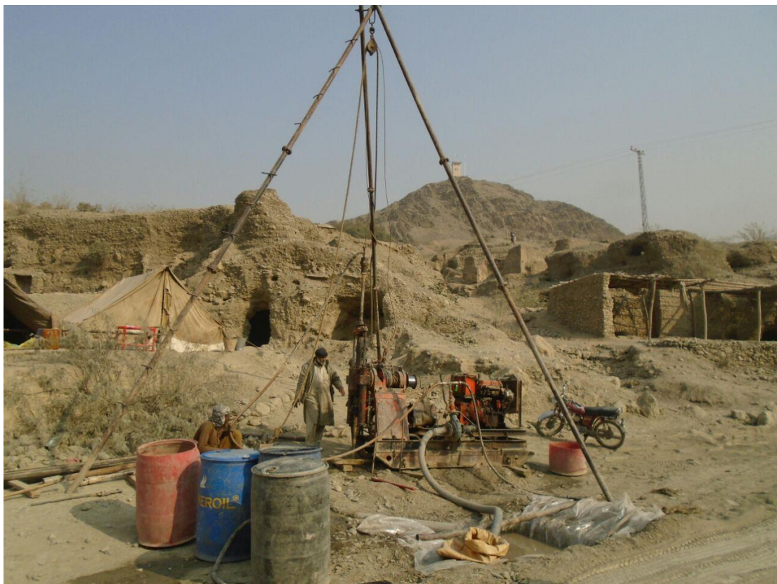
Geotechnical Investigations at Torkham Border, Khyber Agency, KPK
