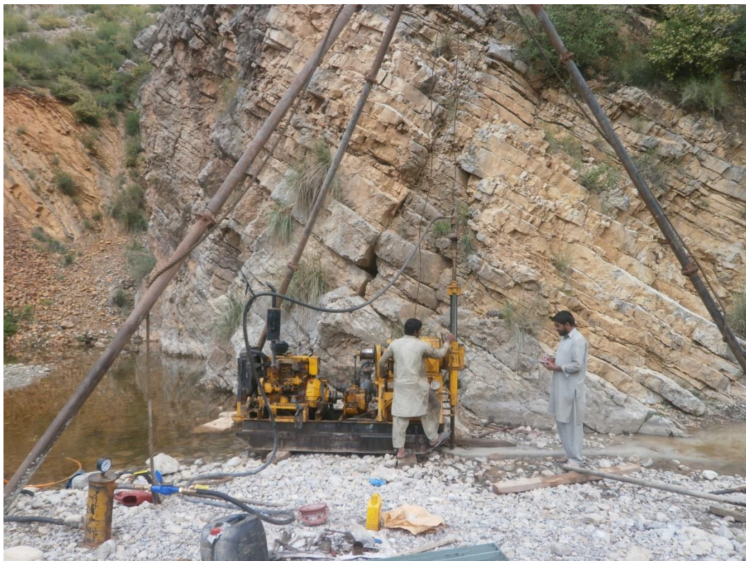
Geotechnical Investigations of Marobi Dam, District Nowshehra, KPK
