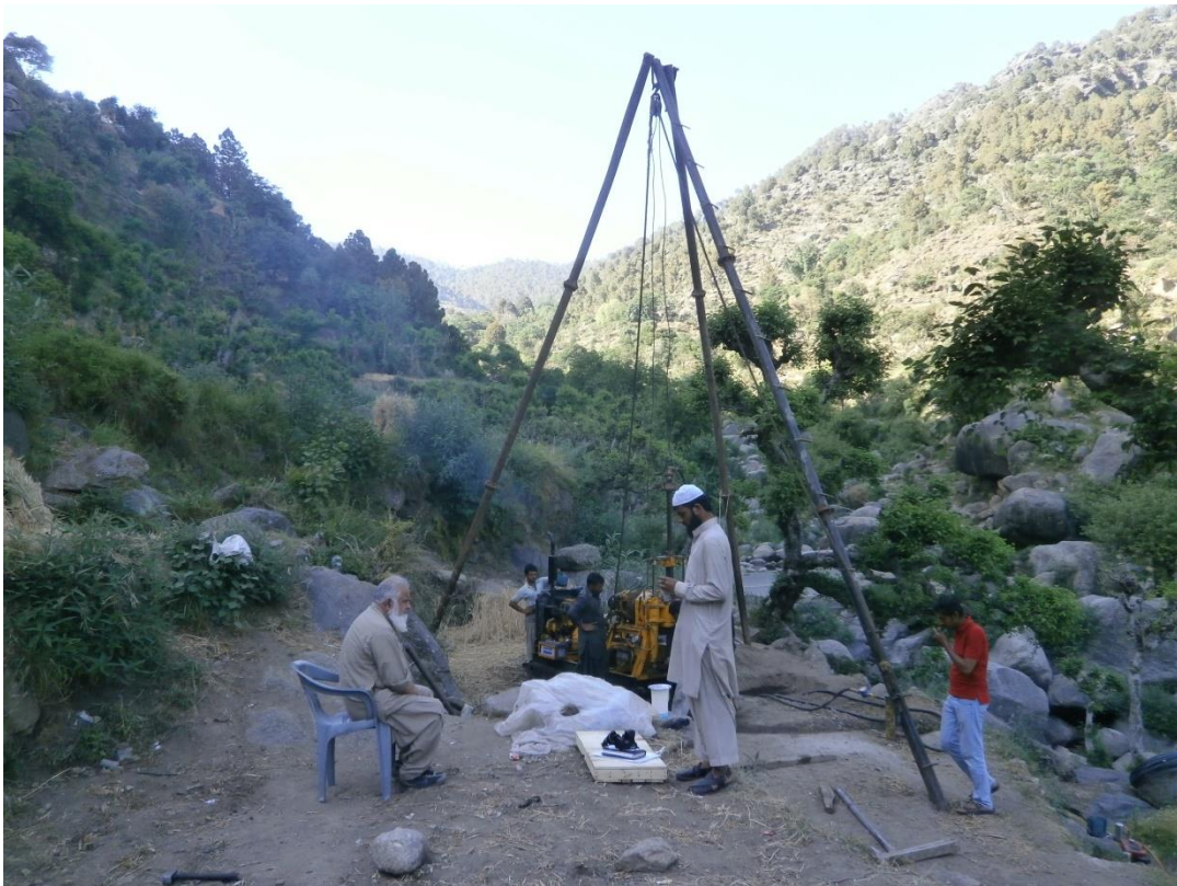
Geotechnical Investigations of Uvla Dam, District Swabi, KPK
